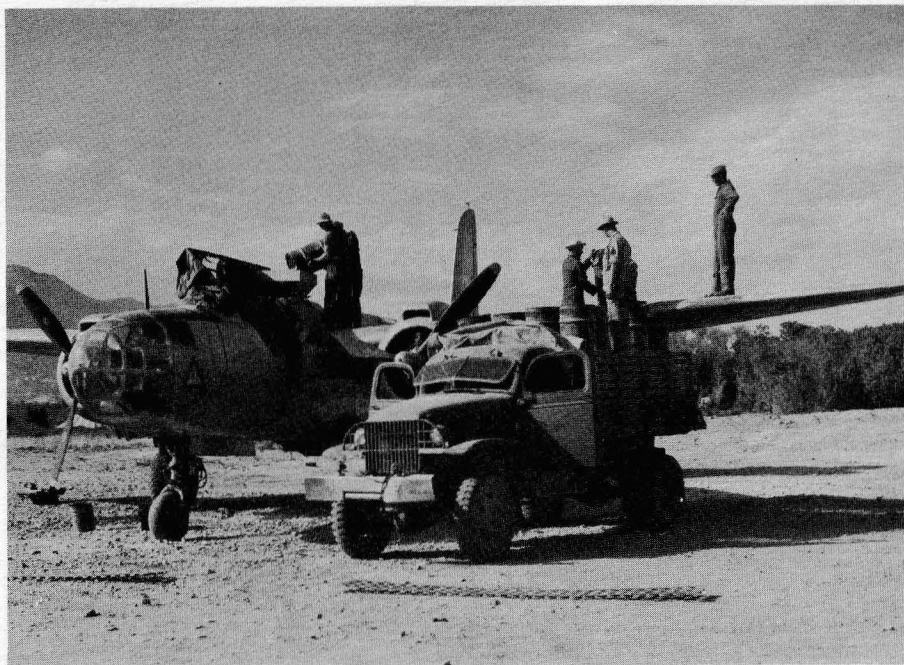
Ground crew members load Paris Green and lime dust into hopper of this A-20 for aerial mosquito spray. Corsica
